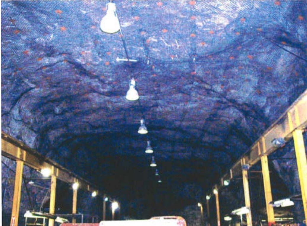
Figure 16.9: 2,500 Level Shop Ground Conditions
