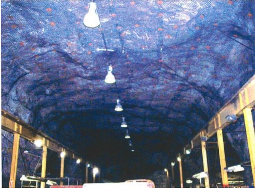
Figure 16-9: 2,500 Level Shop Ground Conditions
