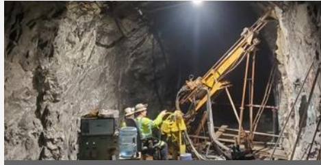
Underground Drilling at ESM
