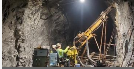
Underground Drilling at ESM
